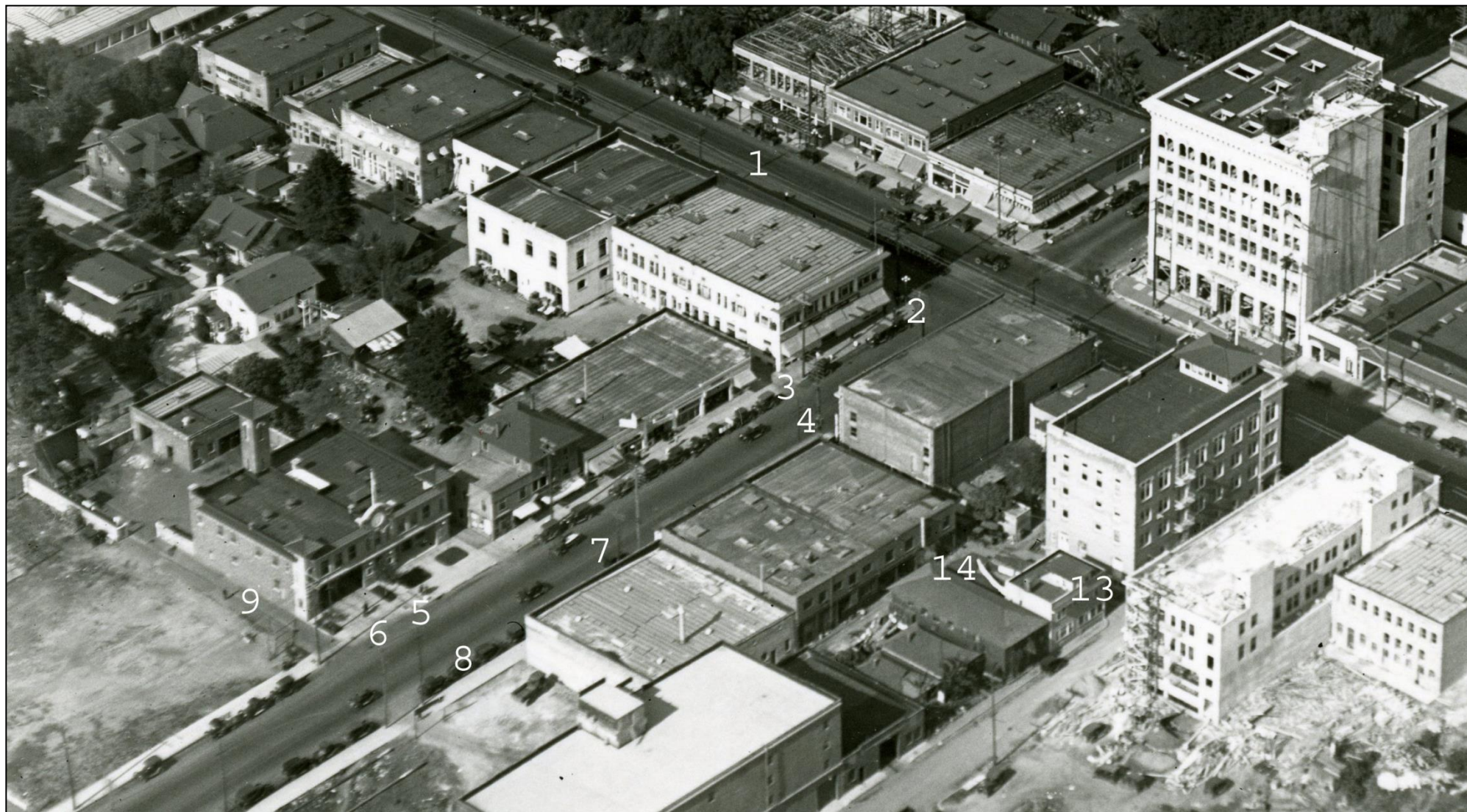
Looking NW at Cahuenga running from lower left towards Hollywood Blvd., with numbered tour highlights. Notice the vacant lots at lower left. The Chaplin-Keaton-Lloyd Alley runs from 4 past 14 to 13.
